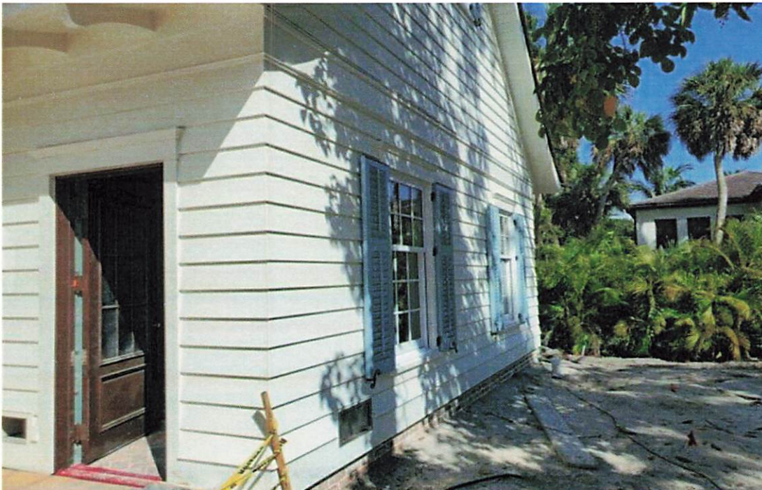
RIGHT SIDE GARAGE, 6/6/2023
