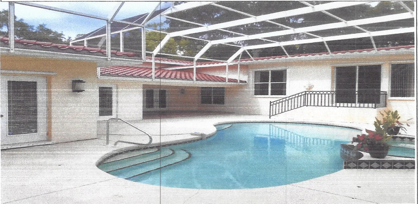
Photo Two Caption 1332 Quail Drive - Rear Photo
