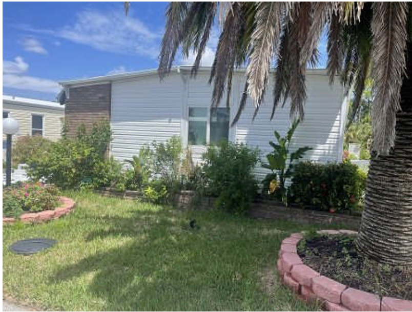
Photo One Caption: FRONT VIEW 08/28/2024 Clear Photo One
