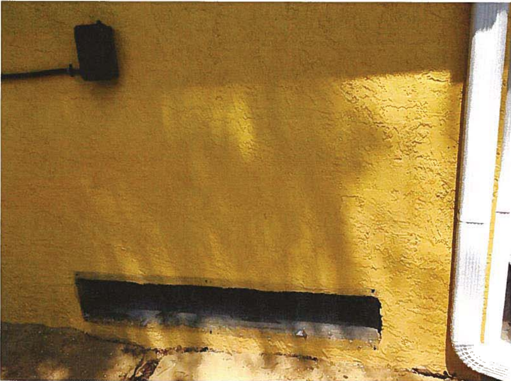
Styrofoam removed from flow through openings.
