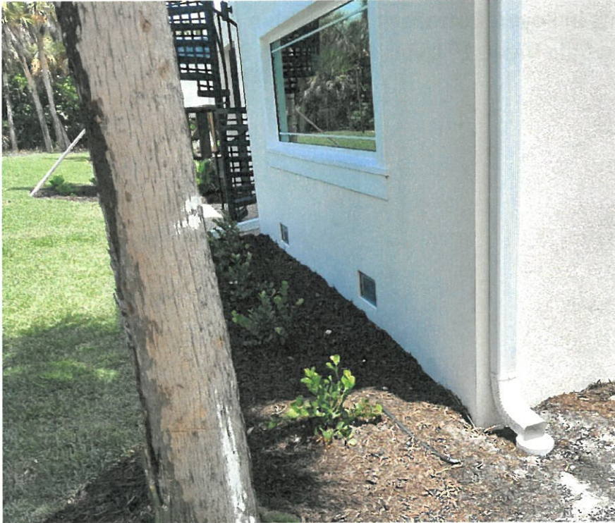
(06/13/2024) Rear Structure Wall, Left Side Garage/Storage, 2 Smart Vents Total of 16 Smart Vents in Rear of Structure Walls.
