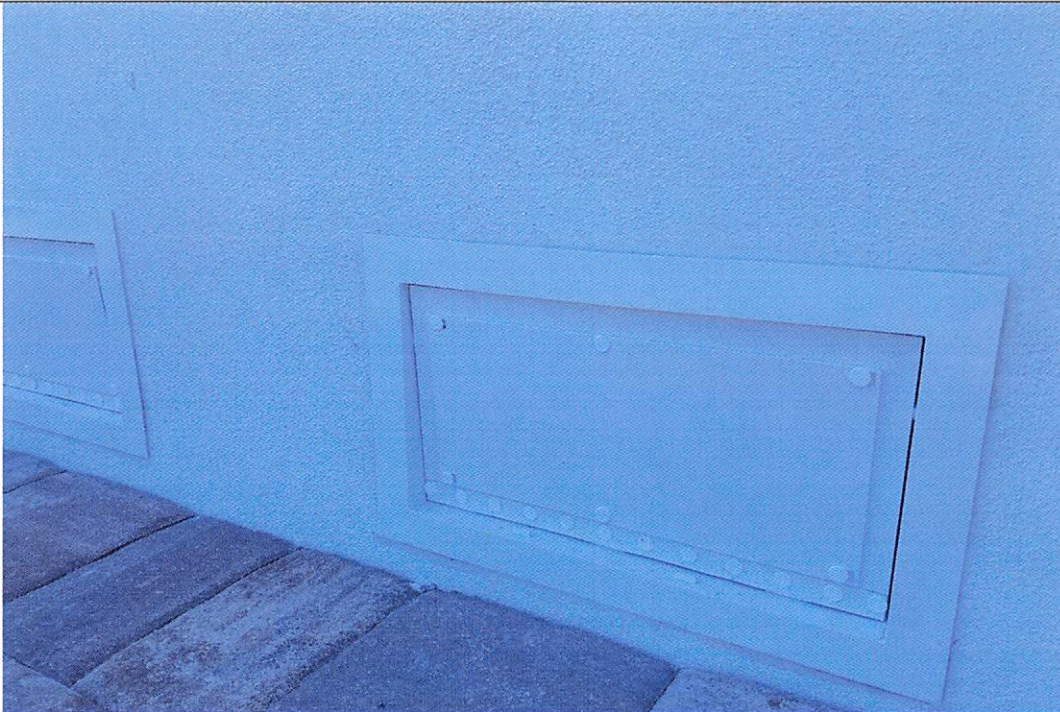
(Typ) Garage wall Flood Vents
