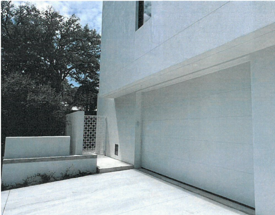
(04/18/2024) 2 Smart Vents in Parking Area East Wall
