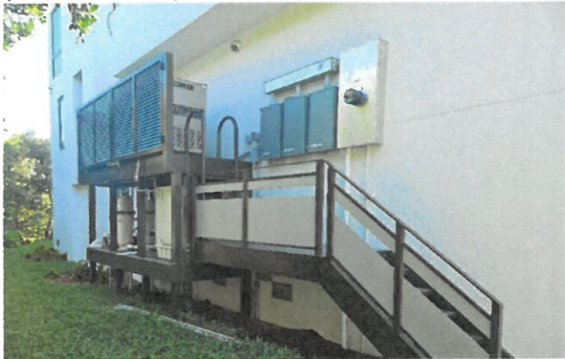
(04/18/2025) Elevated AC Unit & Generator on Platform= 11.9'.
