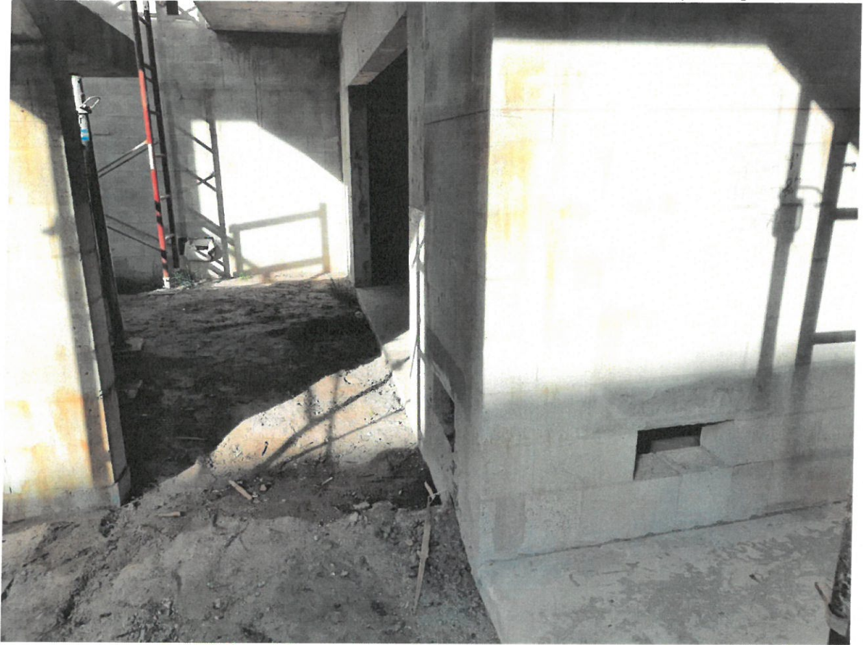
(04/10/2023) Front/Side View of 2 Storage Areas with 3 Flood Openings Total
