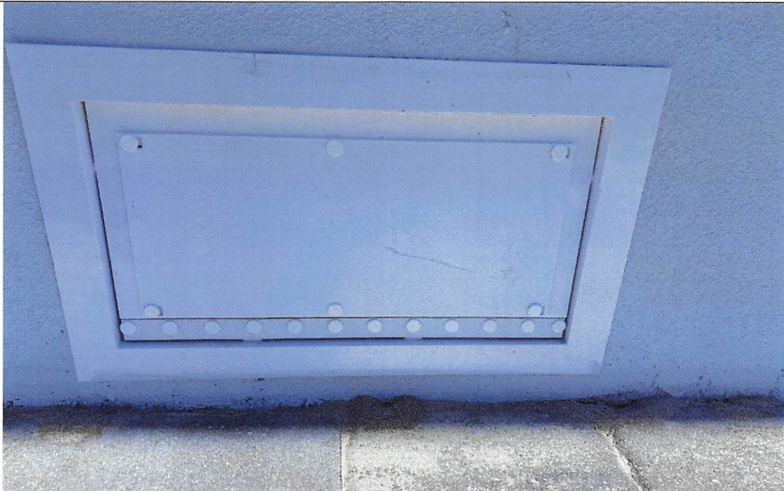
Photo 5 Caption (Typ) Garage wall Flood Vents JOB# 18-1485 Date Taken 2/25/21
