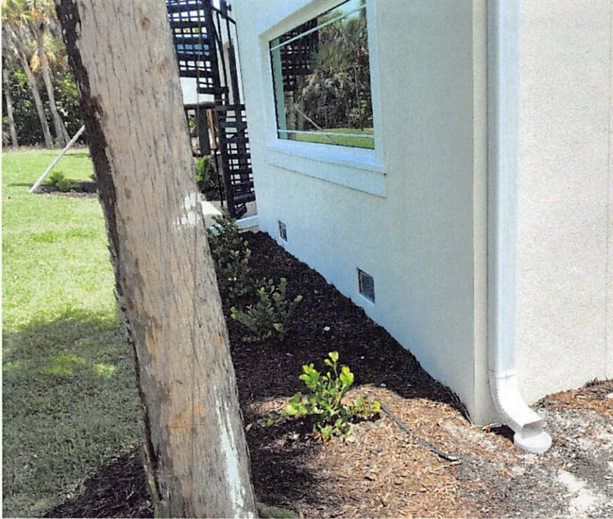
(06/13/2024) Rear Structure Wall, Left Side Garage/Storage, 2 Smart Vents Total of 16 Smart Vents in Rear of Structure Walls.
