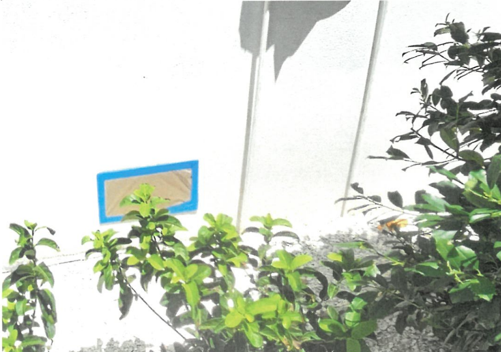
(08/08/2025) 1 Flood Flap Flood Vents in Left Side Wall of 1 Car Garage
