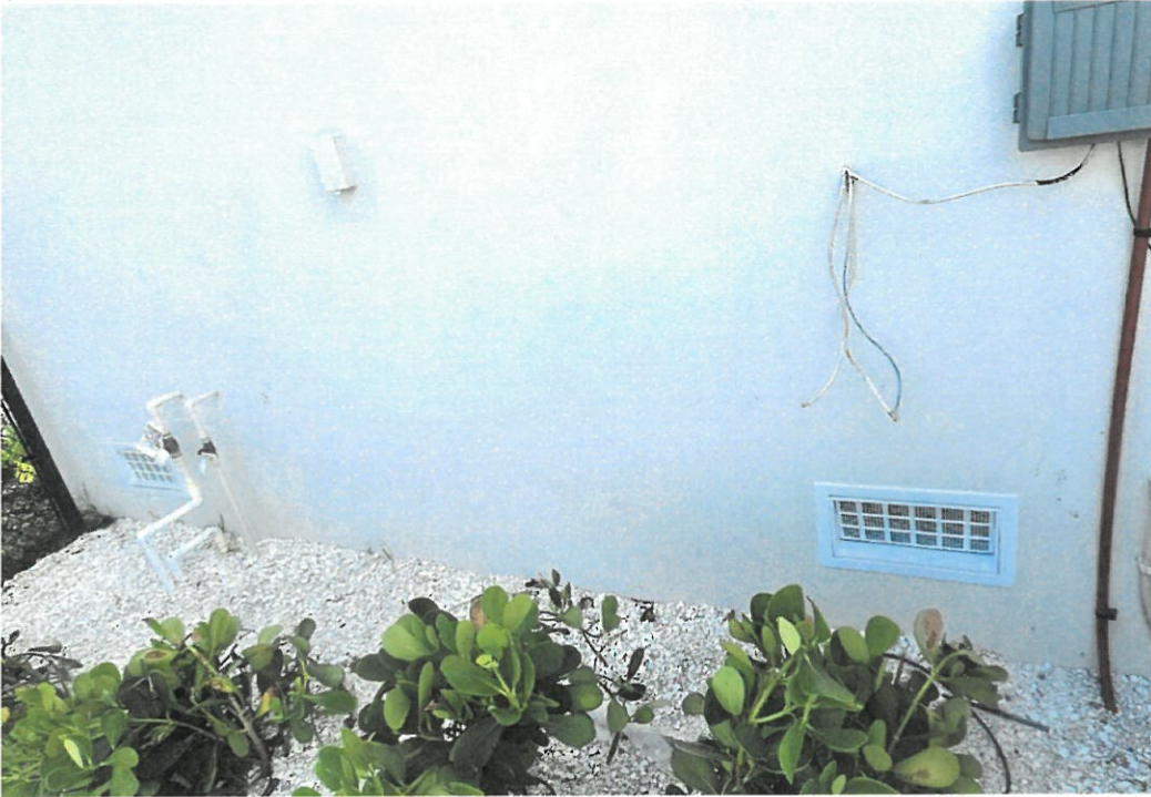
(08/08/2025) 2 Flood Flap Flood Vents in Right Side Wall of 2 Car Garage
