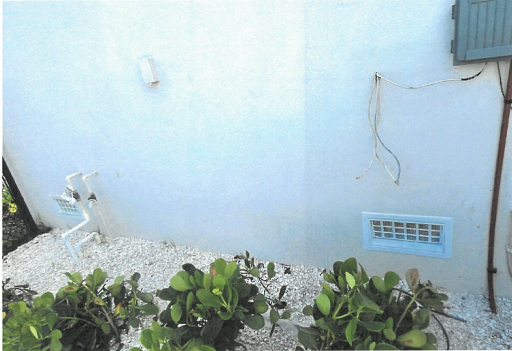
(08/08/2025) 2 Flood Flap Vents in Right Side Wall of 2 Car Garage
