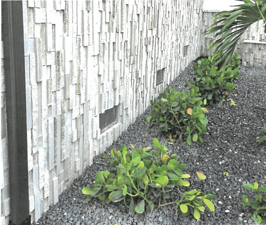
(08/13/2025) 3 Smart Vents Model #1540-520 on Right Side Wall of Garages
