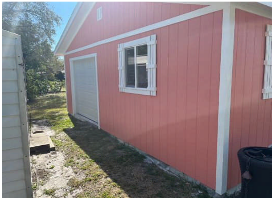
Photo Two Caption: REAR VIEW 02/27/2024
