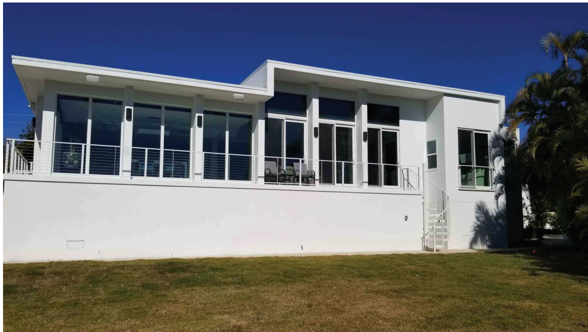
Photo Two Caption: REAR VIEW 02/10/2026
