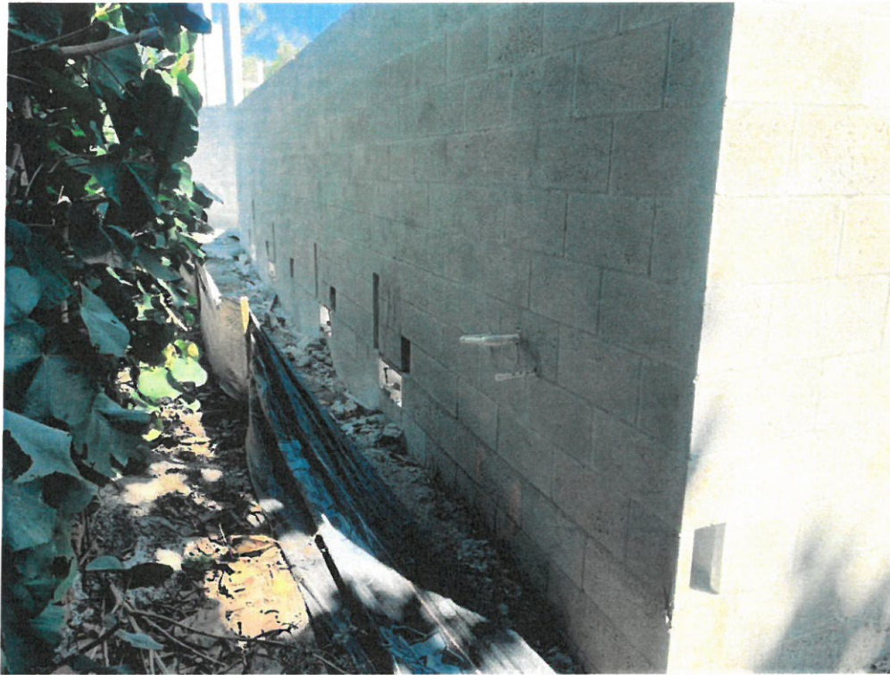
(02/20/2023) Left Side View from Front, 4 Flood Openings in Garage Wall
