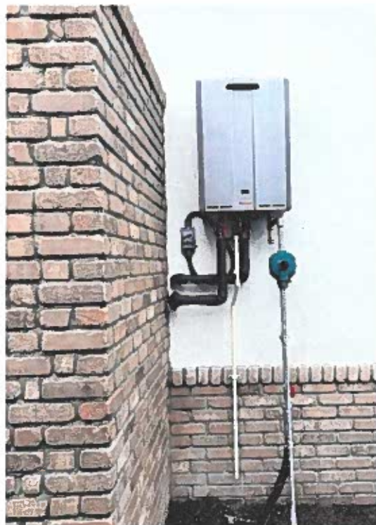
(03/03/2023) Tankless Water Heater Inside Garage on Wall & on Outside Wall
