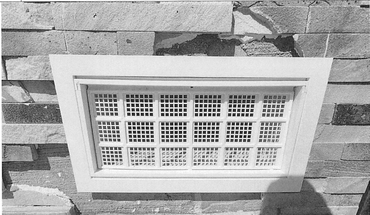
Photo 6 Caption Individual Vent Detail JOB# 17-1531 Date Taken 5/31/23
