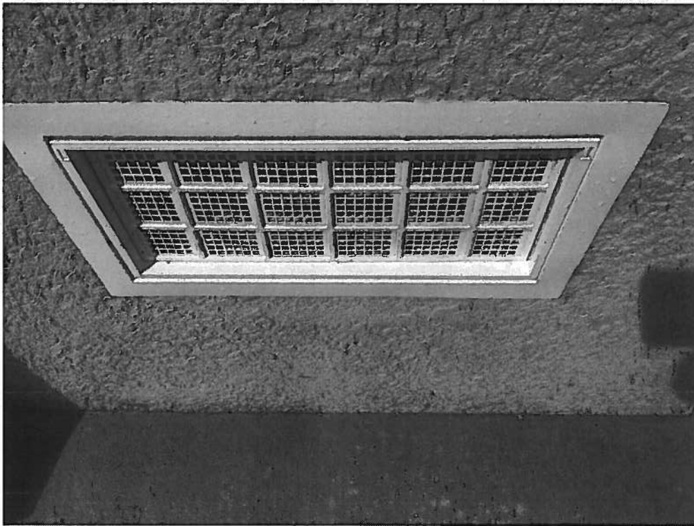
Close up of vents installed over all 4 openings.
