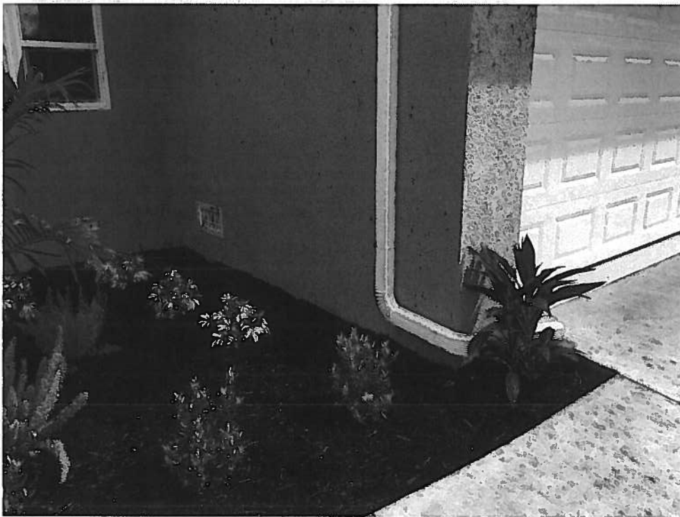
1 vent installed on opposite wall.
