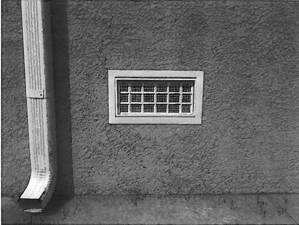
Close up of vents installed over all 4 openings.
