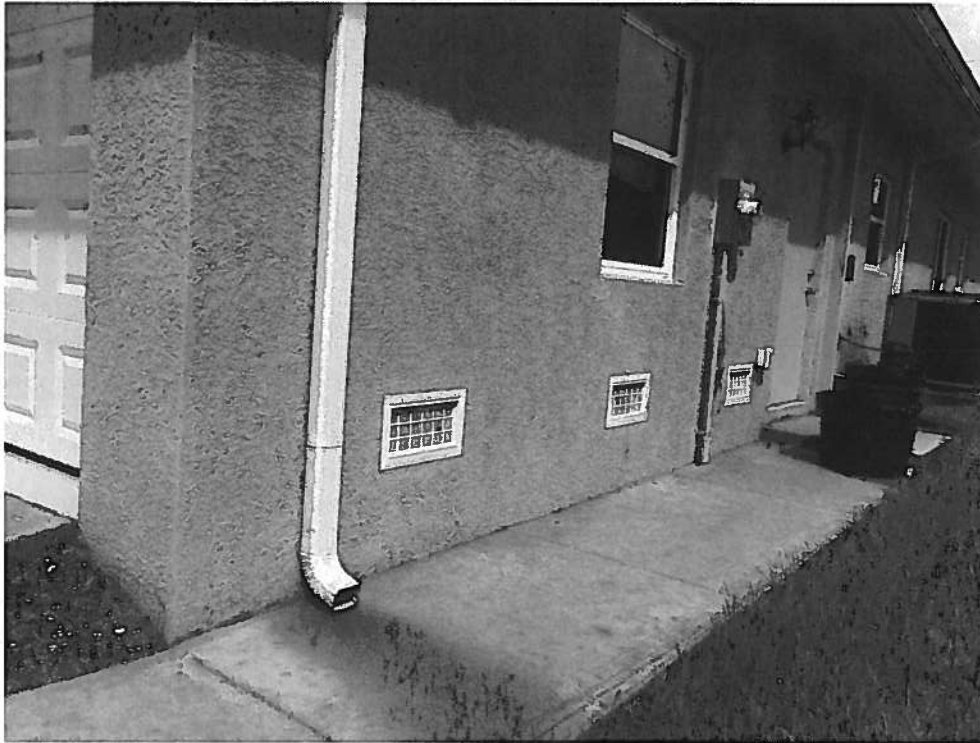
3 vents installed on one side of garage.
