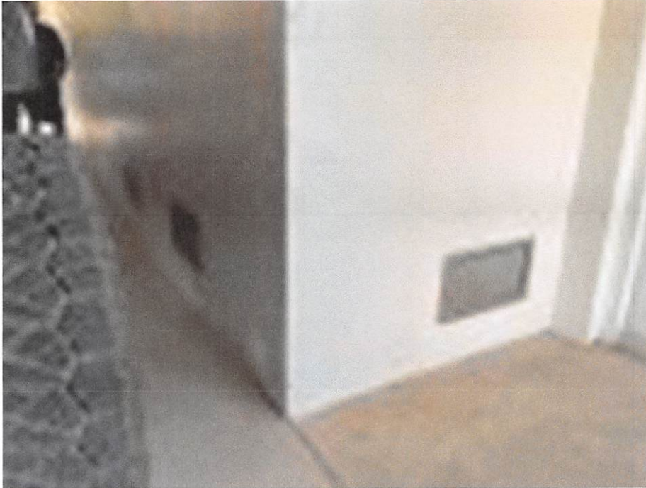
Photo Caption: 05-23-2023, FLOW THROUGH PARTIALLY ENCLOSED AREA 2
