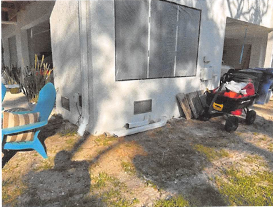
Photo Caption: 05-23-2023, FRONT RIGHT STORAGE AREA
