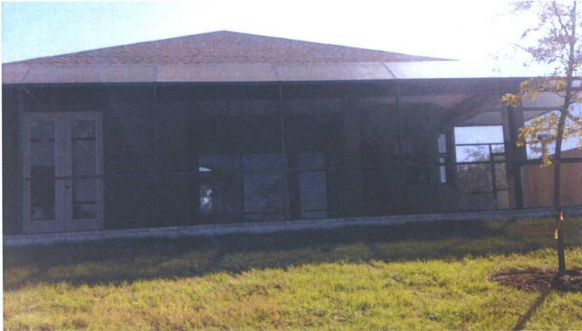
REAR OF HOUSE LOOKING EAST:
