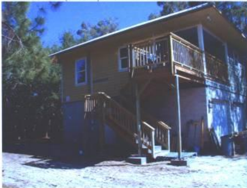
FIGURE 1: (04/03/12) FRONT/LEFT SIDE ENTRY VIEW
