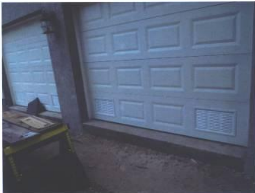
FIGURE 4: (04/20/12) 4 FLOOD VENTS IN GARAGE DOORS VIEW
