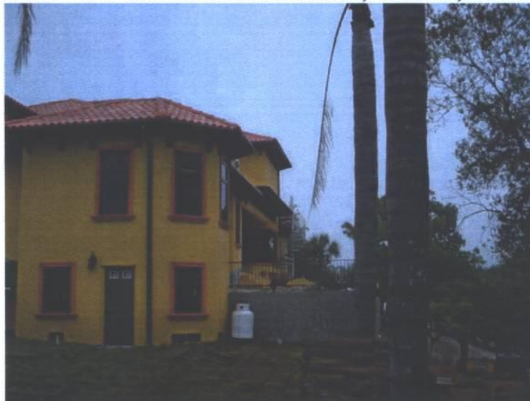
RIGHT REAR VIEW AT 205 BECKER ROAD, VENICE, FL 34293
