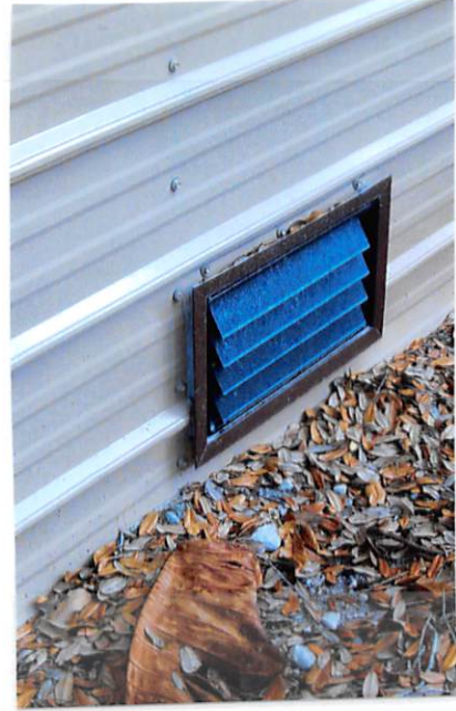
VENT ON SOUTH SIDE
