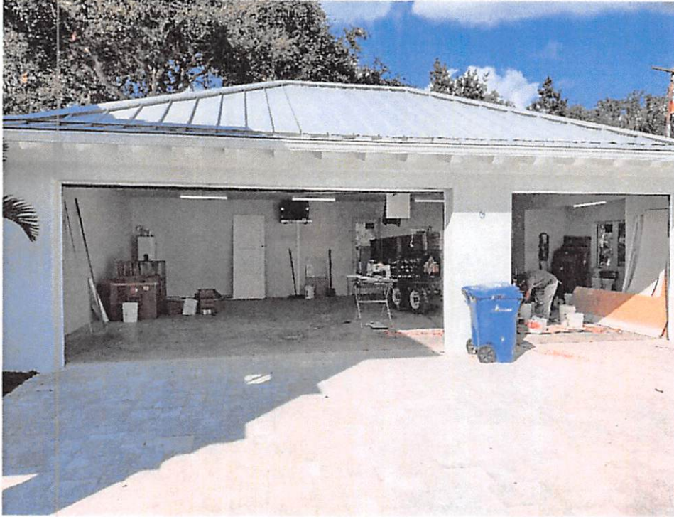
(11/02/2021) Tank Less Hot Water Heater on Rear Garage Wall
