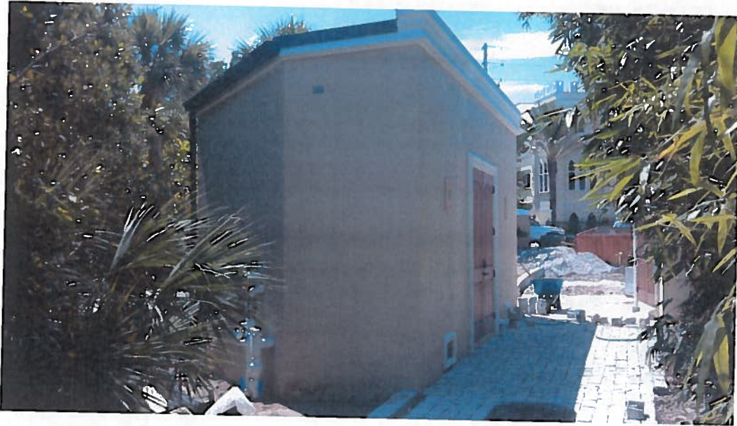
9/04/2012 "Front View" (North)
