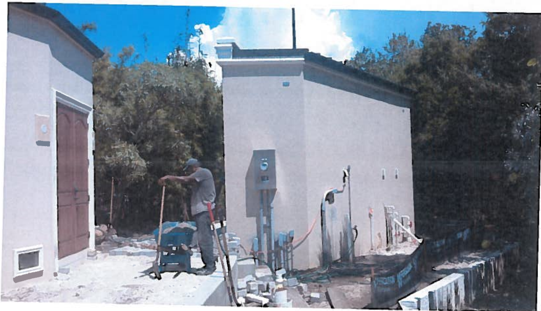
9/04/2012 "Side View" (West)
