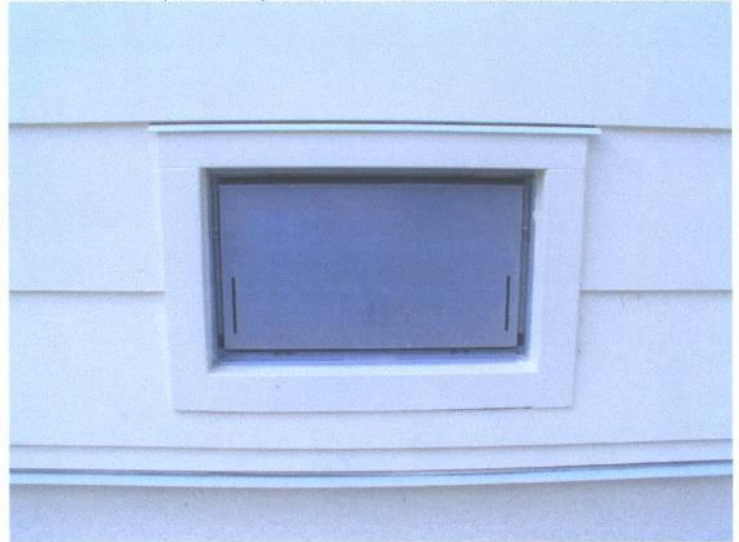
FIGURE 5: (11/04/13) VIEW OF FLOW THRU SMART VENTS
