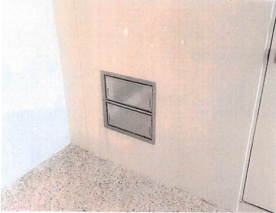
(12/02/2021) Typical Double Smart Vent Model #1540-520
