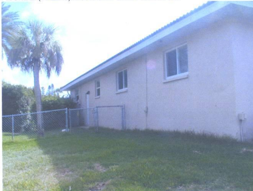
FIGURE 2: (11/22/13) RIGHT SIDE VIEW FROM REAR
