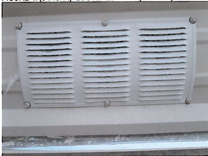
FIGURE 4: (04/15/14) LOUVERED VENT (12 EACH)
