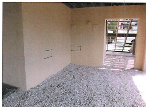
VENT NOT INSTALLED 8-1-14
