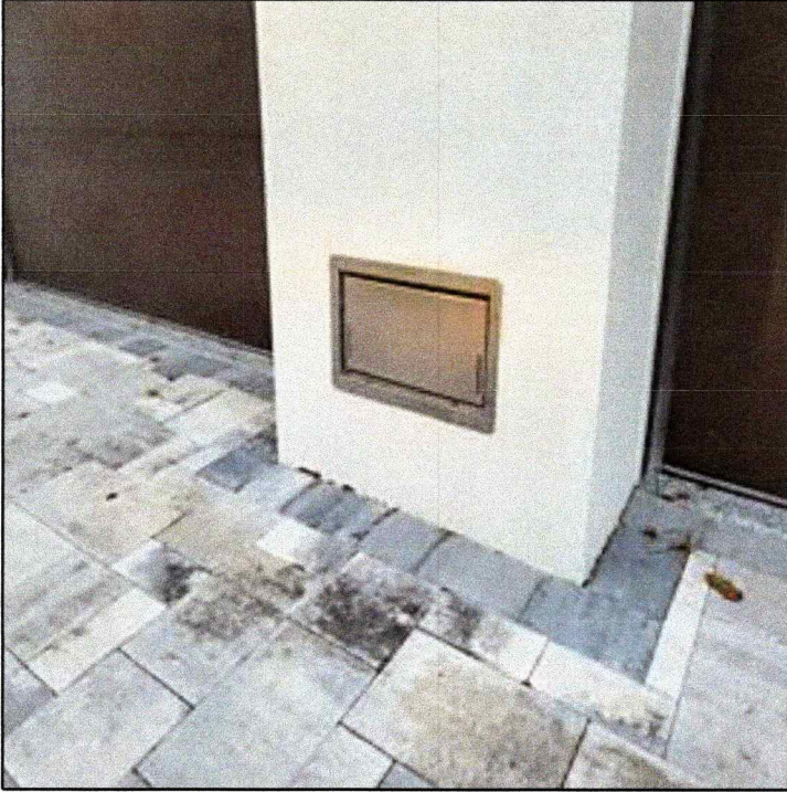
VENT PHOTO TAKEN ON DECEMBER 11 2024
