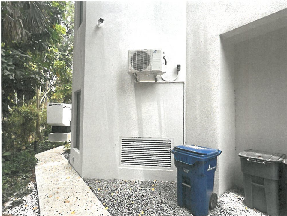
(05/24/2024) Non-Engineered Flood Vent on Rear Wall of Parking Area with Elevated Wall Mounted AC Unit, Elevation = 14.1.
