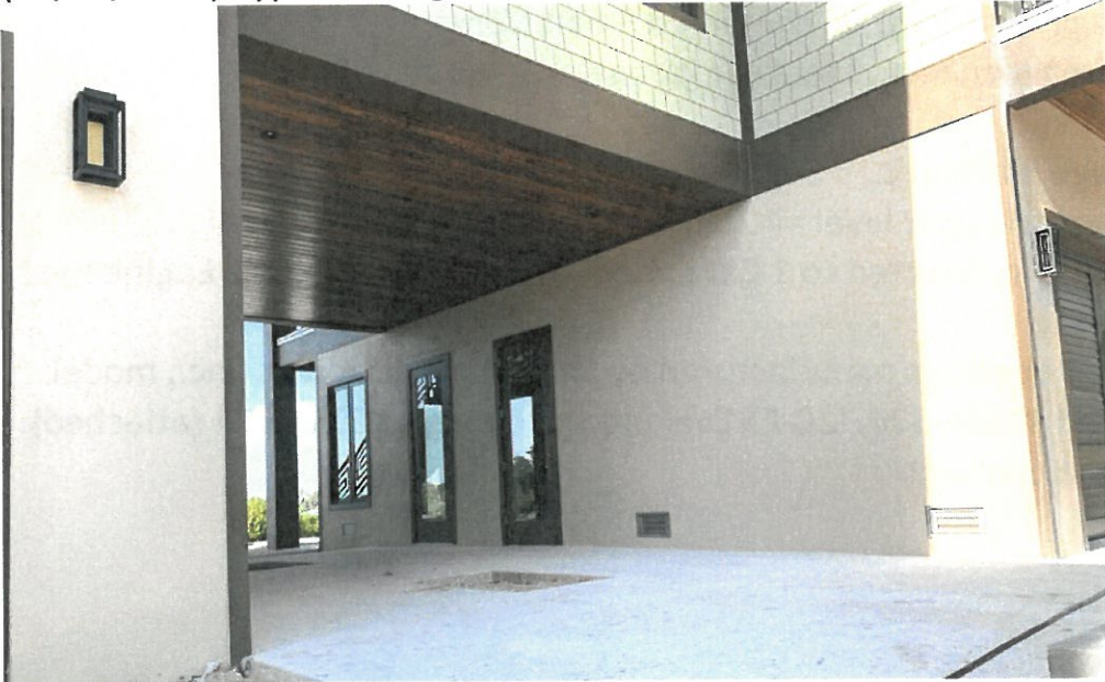
(04/09/2024) Typical 3 Engineered Smart Vent in Breezeway from Front
