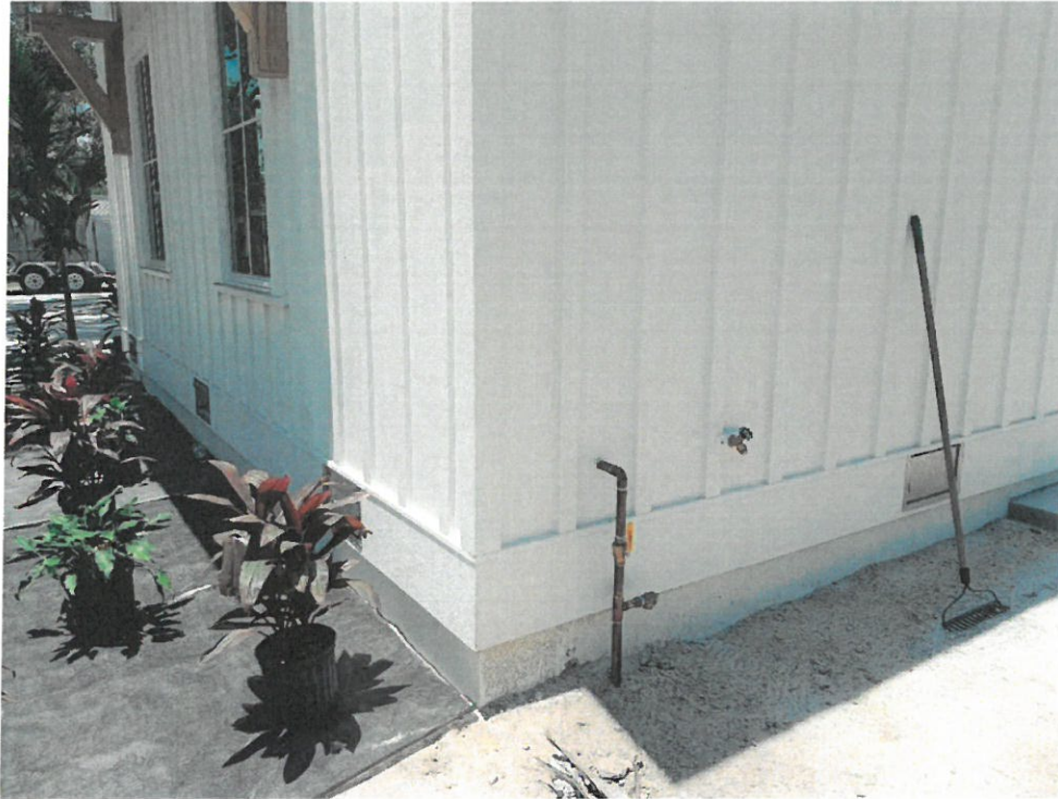
(06/14/2023) 4 Smart Vent Model #1540-570 in Garage Walls
