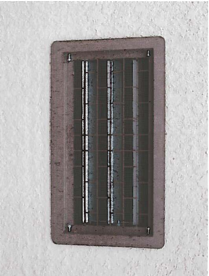
Photo Four Engineered Flood Opening
