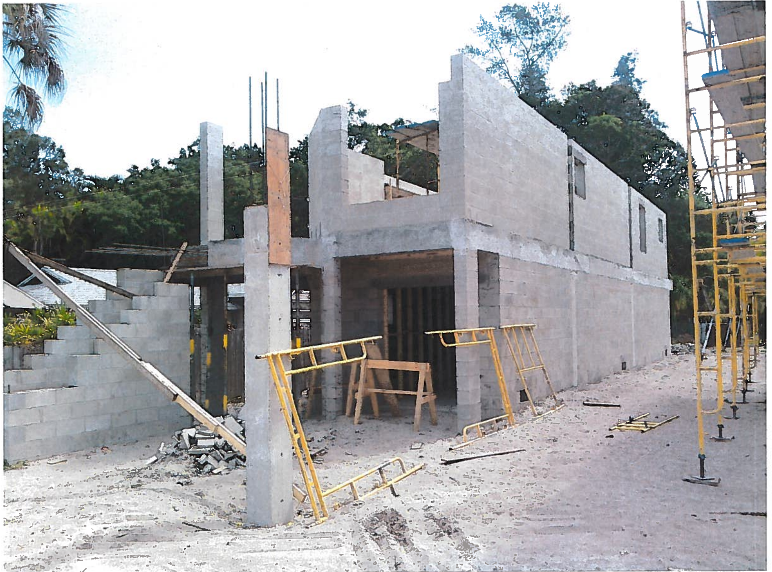
EXHIBIT 1: (4-22-16) WEST AND NORTH SIDE VIEW
