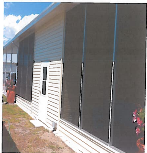
REAR VIEW OF ATTACHED SHED 5-11-2012
