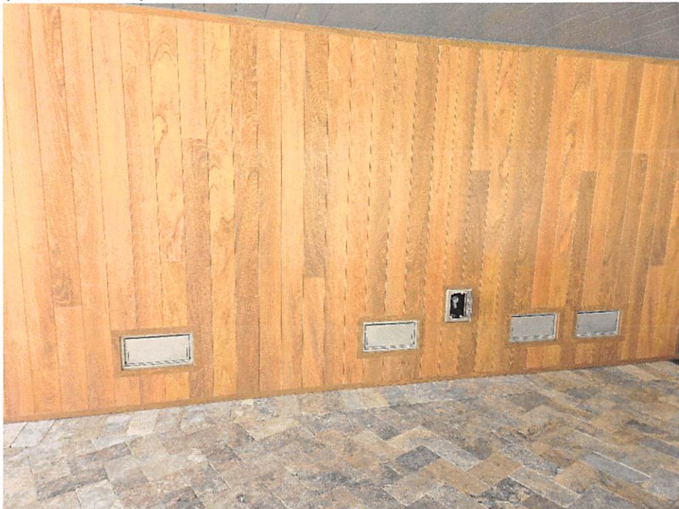
(09/04/2024) 4 Smart Vents on Rear of Structure Under Covered Area
