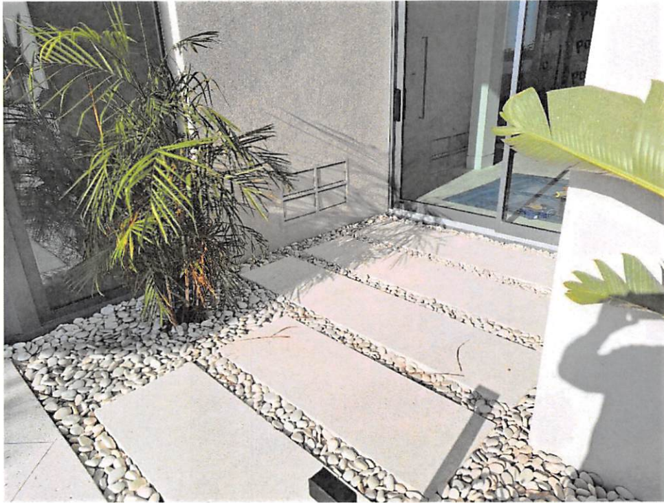
(05/24/2024) 4 Smart Vent Model #1540-520 on Left Side Wall of Small Storage.
