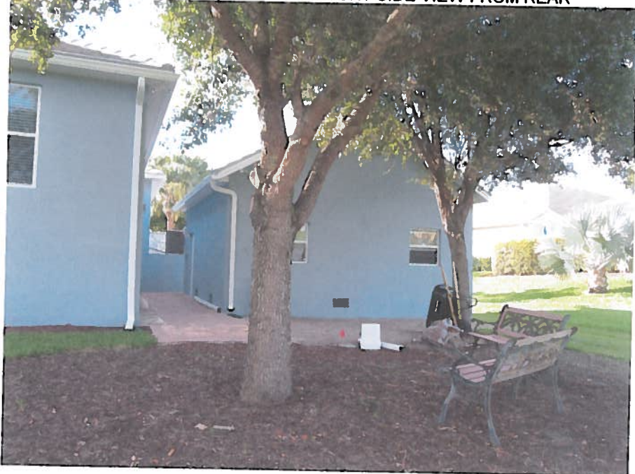
FIGURE 3: (07/08/14) REAR AND RIGHT SIDE VIEW FROM REAR
