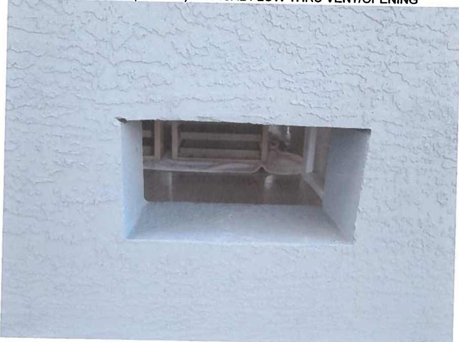
FIGURE 4: (07/08/14) TYPICAL FLOW THRU VENT/OPENING
