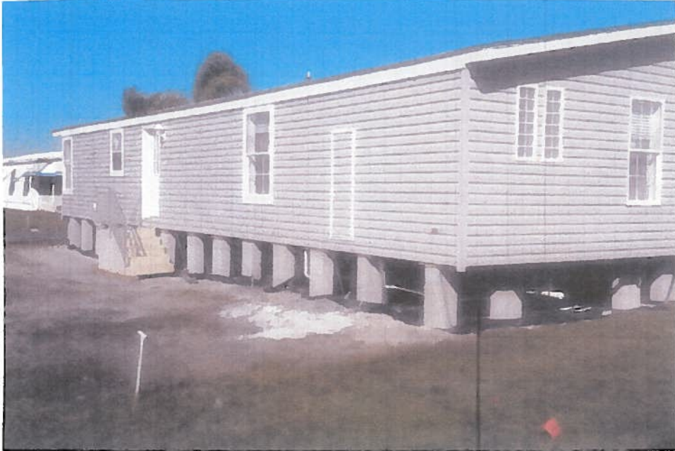
WEST SIDE VIEW
