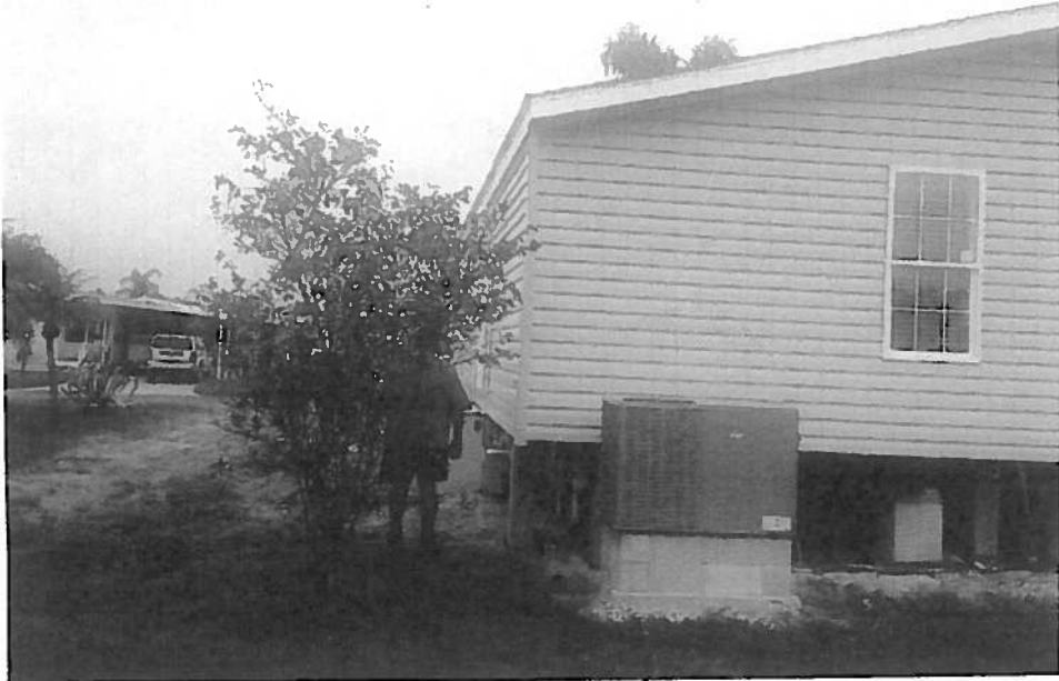
WEST SIDE VIEW
