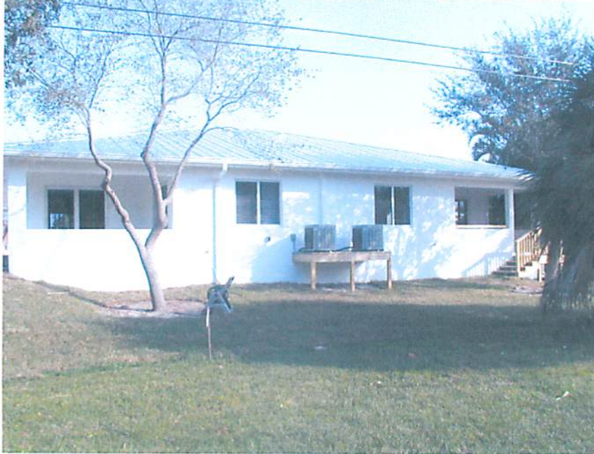
FIGURE 3: (02/13/13) REAR VIEW WITH RAISED AC PLATFORM
