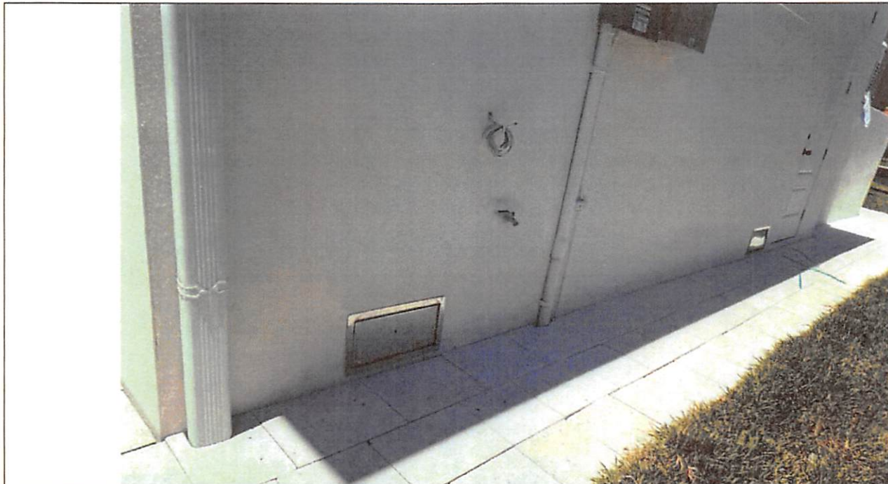
Photo 5 Caption Typical Garage Door Vent JOB# 20-1466 Date Taken 5/15/23
