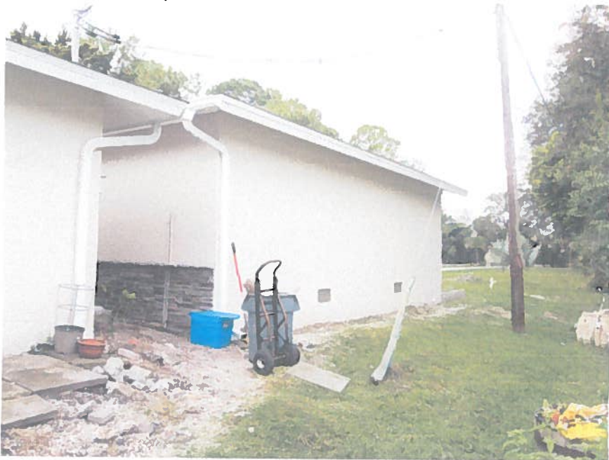
FIGURE 3: (09/10/15) REAR & RIGHT SIDE VIEW
