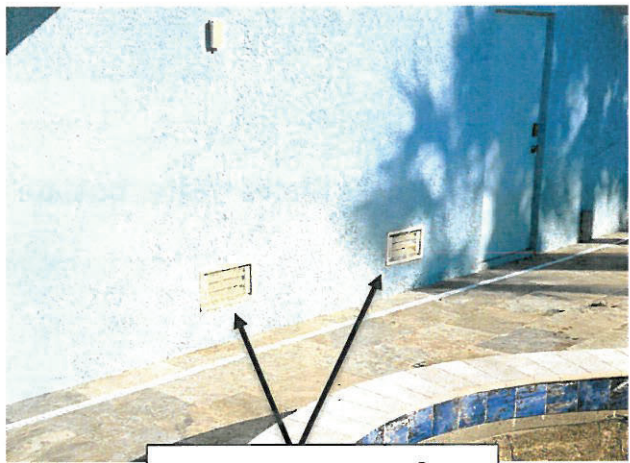
Garage A - Vents #6 & #7
