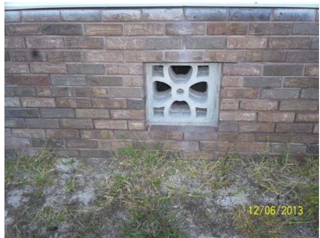
CRAWL SPACE VENT
