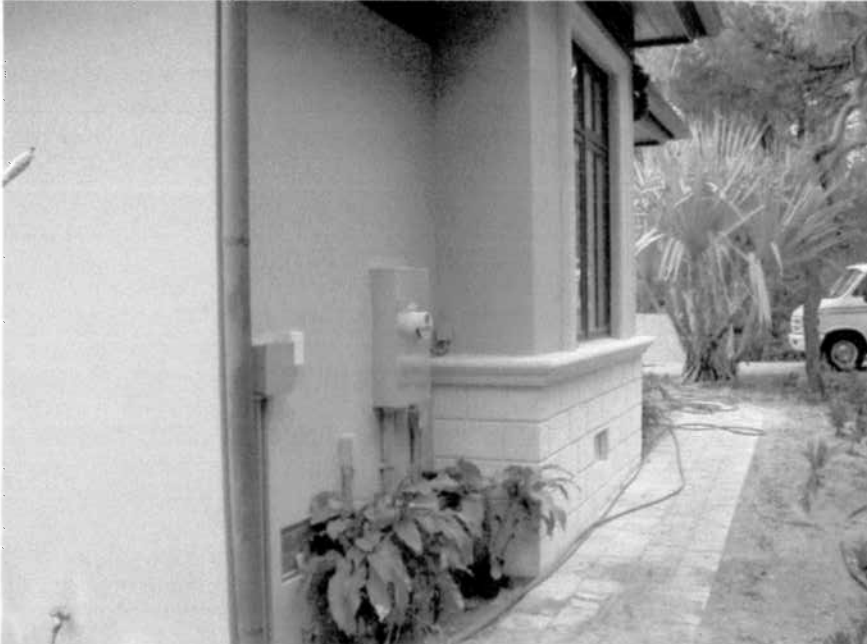
FIGURE 2: (03/13/13) RIGHT SIDE VIEW FROM REAR
